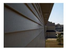
• Monitor: The siding is buckled at the upper west side of the home. Adjustment may be needed.
