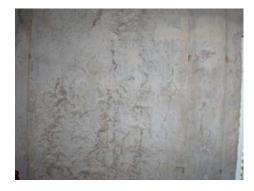
• Monitor: Cold joints/cold pour were observed in the foundation walls. (Dark lines in the concrete or exposed stone) These are caused by the first concrete poor starting to take a set before the second load was poured. This is not a structural concern. In rare cases some seepage could occur along the joint or where stones are exposed.
